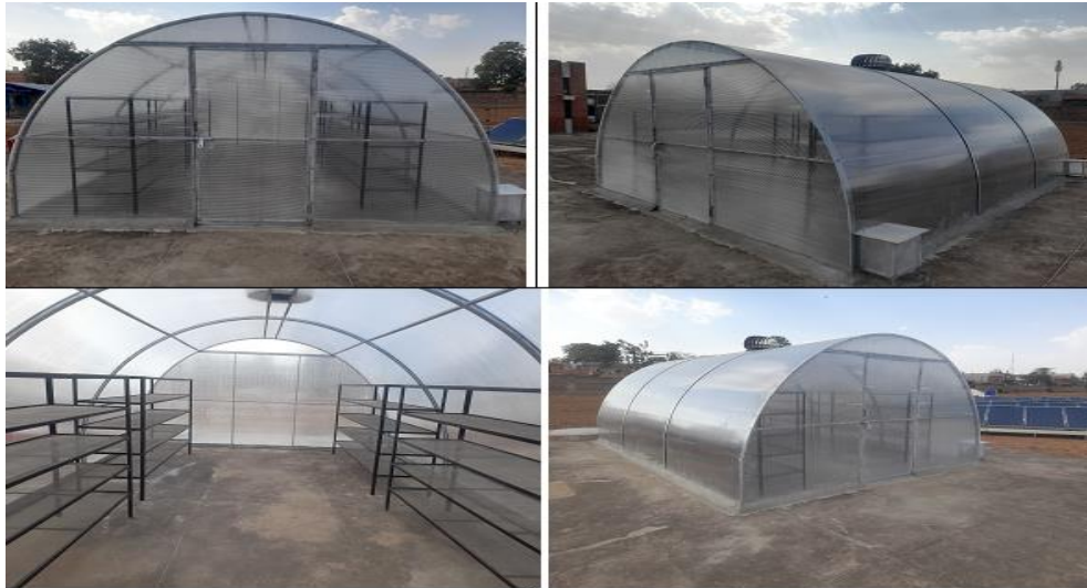
Fig. 2 Actual installation of large-size tunnel-type PV/thermal hybrid solar dryer at solar yard
