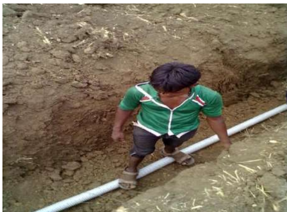
Installation of sub surface drainage
