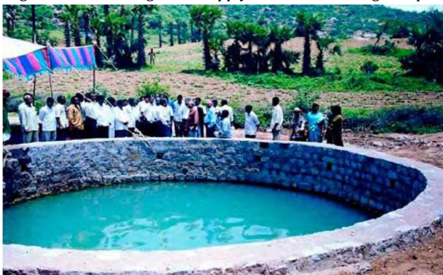
Capture well rejuvenated by recharged water
