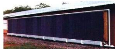
Cooling livestock buildings by Pad and Fan Evaporative Cooling System (Pad Cooling)
